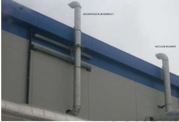
d. Advantage run exhaust ve vacuum blower bacası
